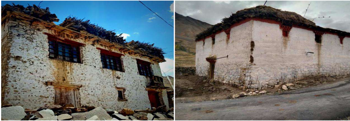
Dry stone construction
