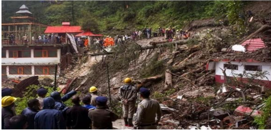
Figure 5 Landslide at Shiv Mandir, Summerhill, in Shimla district, Himachal Pradesh
