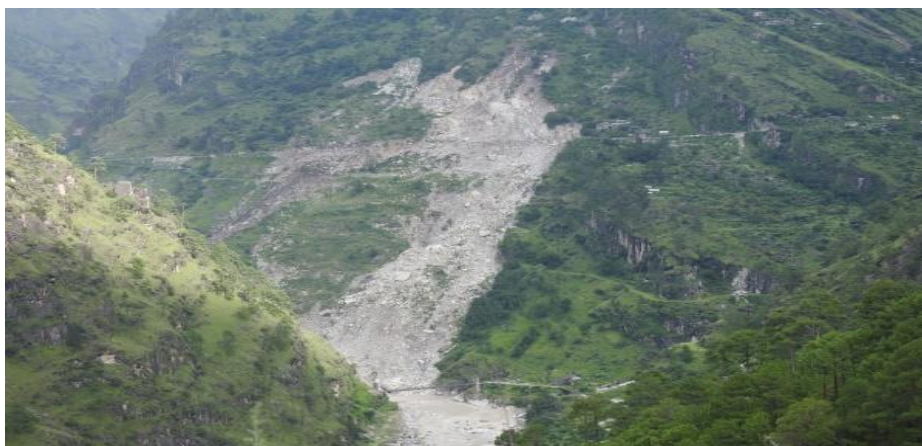
Figure 7 Landslides in Nigulsari, Kinnaur district, Himachal Pradesh
