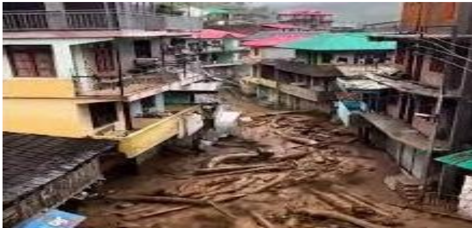
Figure 6 A Flash flood at Thunag Market in Mandi district, Himachal Pradesh
