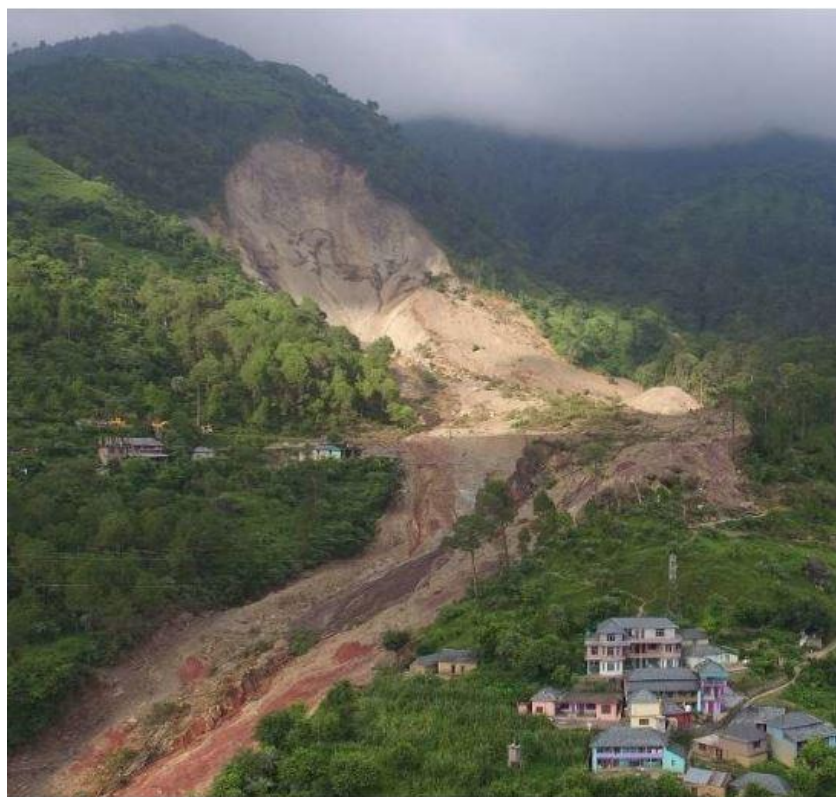
Figure 11 Landslide at Kotropi, Mandi district, Himachal Pradesh (landslide on NH-154, active since 2017, reactivates annually during monsoon)
