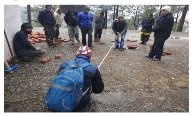
2. Always check dimensions and corners by 3-4-5 method or equal diagonal method.
