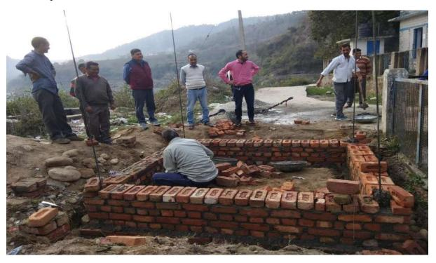
9. Provide RC band and corner steel as per design and detail.
