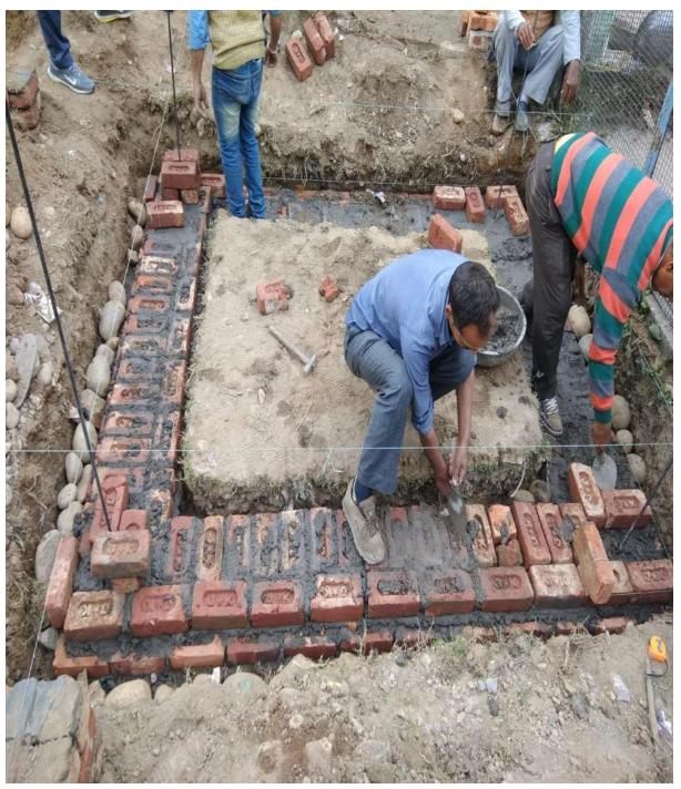
The bar are provided at the corners of walls to make the building earthquake resistant.
