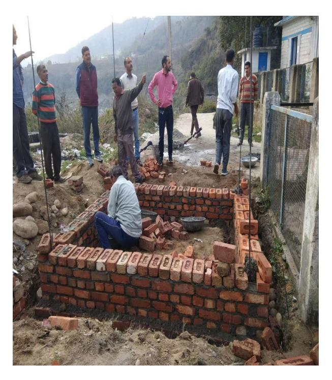
Participants understands how to construct foundations incorporating hazard resistant features. The foundations chosen in these exercises were selected from the locally practiced typologies. Also, participants were exposed to the basics of reinforced concrete footings and details of horizontal bands.
