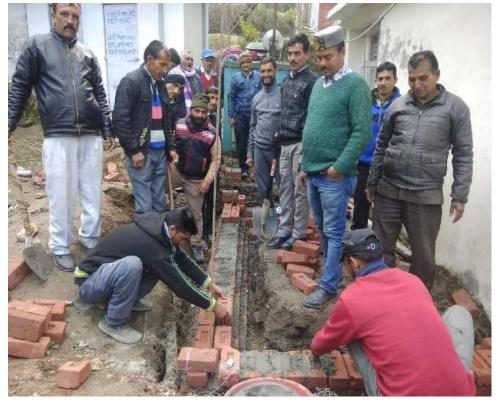
masons are familiar made with the good construction practices, directions of windows, slab thickness, steps to be followed in stone masonry and brick masonry, techniques shuttering, positions of
