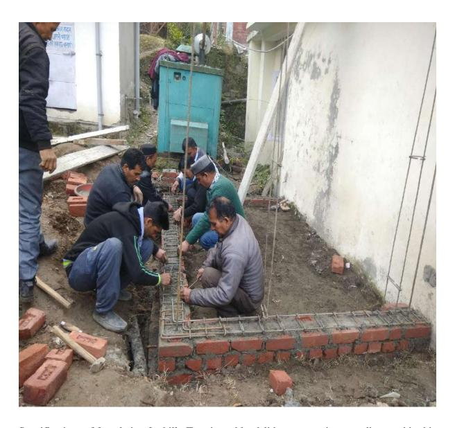
Specifications of foundation for hilly Terrain and landslide prone regions are discussed in this session. Junction of vertical reinforcement and horizontal bands.
