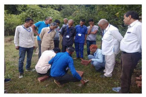
2. Always check dimensions and corners by 3-4-5 method or equal diagonal method.
