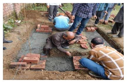
The bar are provided at the corners of walls to make the building earthquake resistant.
