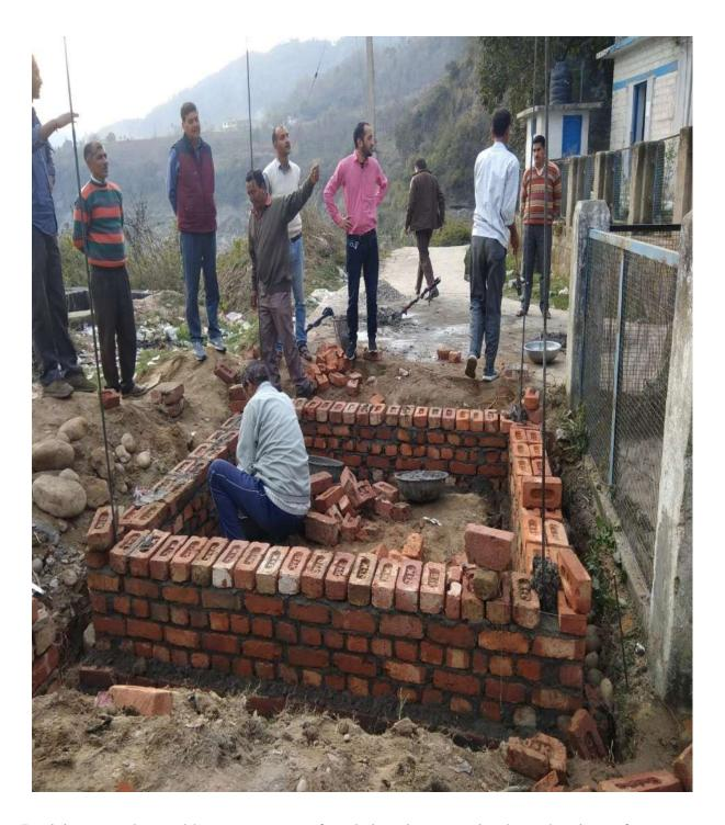
Participants understand how to construct foundations incorporating hazard resistant features. The foundations chosen in these exercises were selected from the locally practiced typologies. Also, participants were exposed to the basics of reinforced concrete footings and details of horizontal bands.
