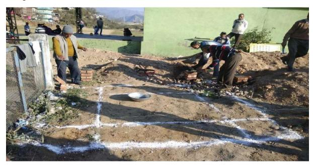
2. Always check dimensions and corners by 3-4-5 method or equal diagonal method.
