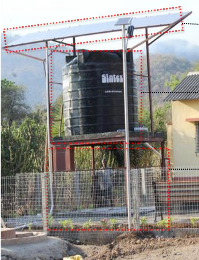
**Solar energy powered** submersible **pump** with required photovoltaic panels
