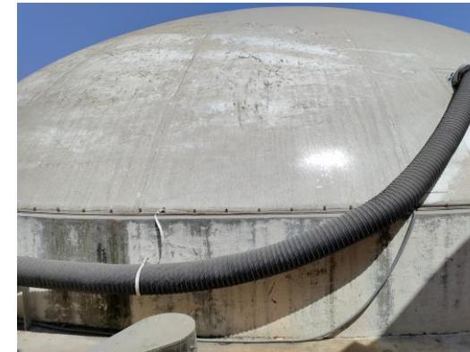
**Methane generated from anaerobic digestion is used for electricity generation (450 KW) and electricity is reused in the STP**
